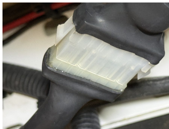
The Molex Mini-Fit Jr junction at the pump control box.
